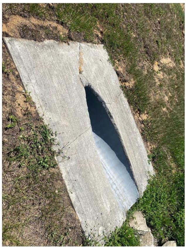
1. POND A1/STORM STRUCTURE 44A-MONITOR CRACKS IN MES
