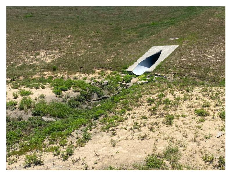
4. STORM STRUCTURE 45B-REPAIR CRACKS/REMOVE DEBRIS & OVERGROWN GRASS FROM MITER END
