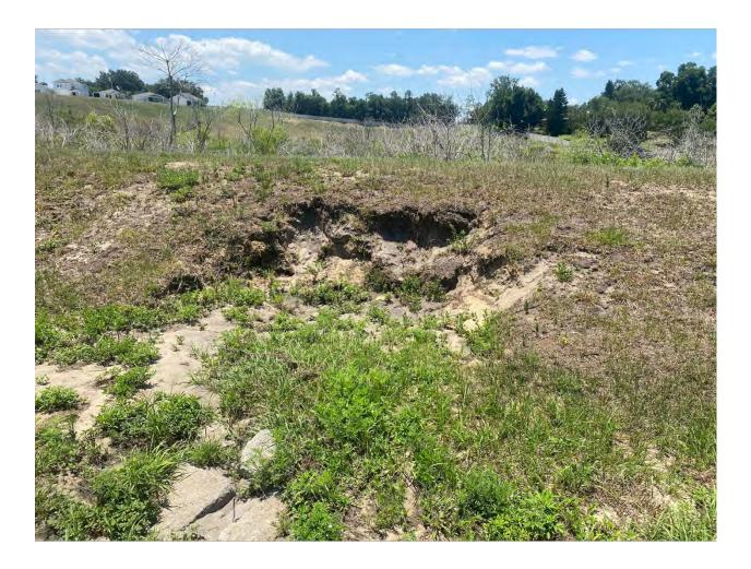
3. STORM STRUCTURE 41B- REGRADE POND BOTTOM, ADD ADDITIONAL RIP RAP AT MITER END
