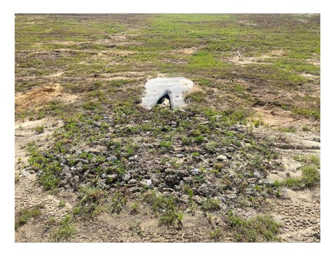
19. TRACT E/POND D STORM 50A – REMOVE DEBRIS/OVERGROWN GRASS FROM MITER END
