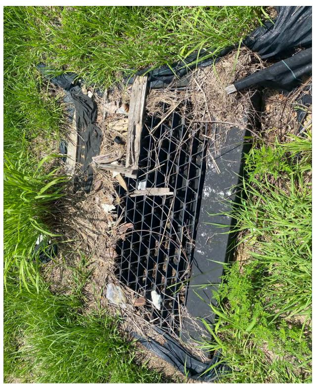
15. SWALE BEHIND LOTS 78-98 LOOKS TO HAVE GRADING ISSUES AND DEBRIS IN STORM 40. WILL NEED TO BE CHECKED AFTER CONSTRUCTION IS COMPLETE.
