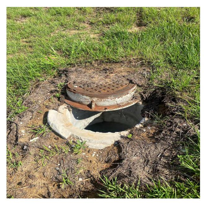
1. STORM MANHOLE 44A – LID HAS SHIFTED OFF STRUCTURE BASE - REPAIR
