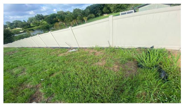
20. THE FENCE ON THE BOUNDARY OF TRACT E IS MISSING MULTIPLE PANELS. THEY NEED TO BE REPLACED.
